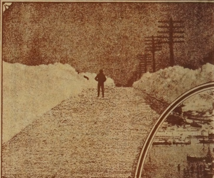
Snow Removal Work on New Jersey Highways keeps the roads open
